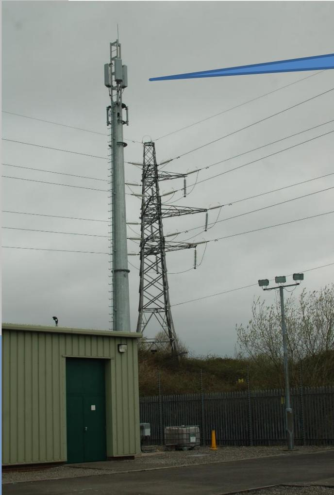
Tri-sector 416 MHz LTE base station mast at Portishead Bulk Supply Point
